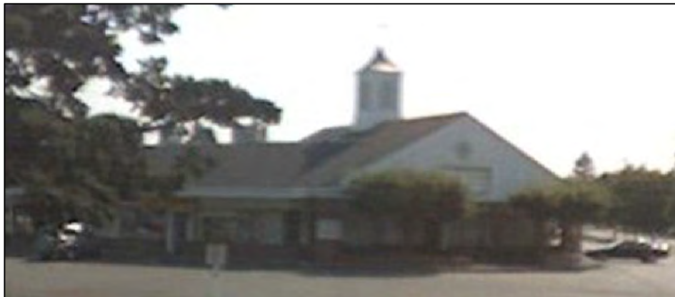
East Building, southwest corner retail (NIC)
