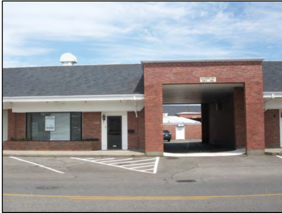
south service drive to inner courtyard (NIC)
