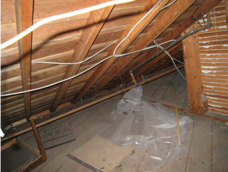
Photo #6 – 1x8 T&G roof sheathing over 2x4 roof joists/rafter
