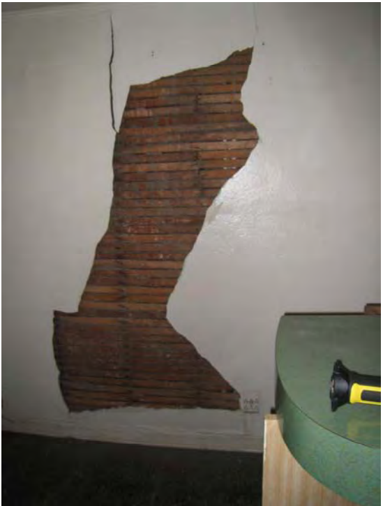
Photo #3 – Lathe & Plaster at interior face of wall
